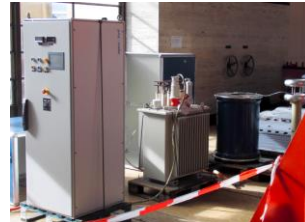
Medium Voltage Test Unit
