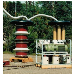
400kV Test Set with MG-Set
